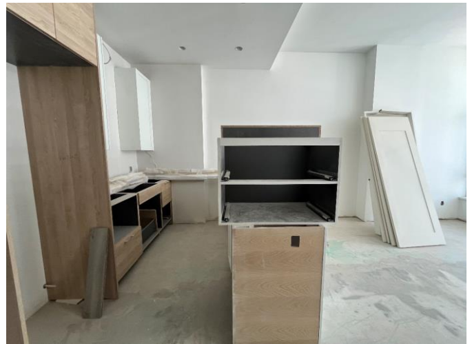
L32 - Cabinetry ongoing
