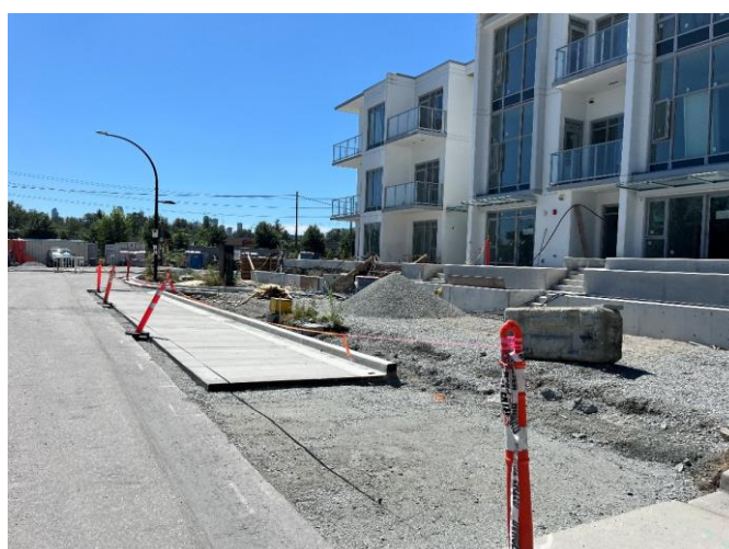
Site works ongoing
