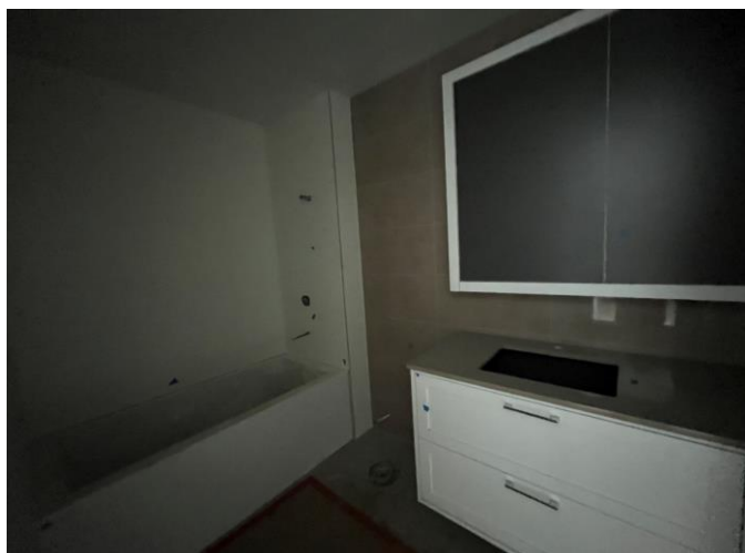
L23 - Bathroom finishes ongoing
