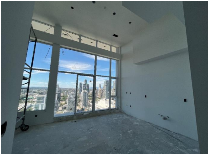
L33 - Prime paint complete
