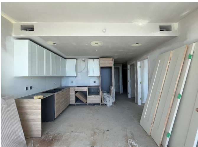
L31 - Cabinetry ongoing and interior doors on site
