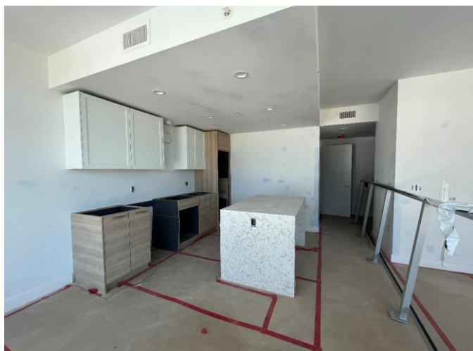
L4 - Balcony rails ongoing
